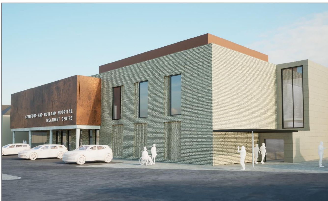
Proposed Day Treatment Centre at Stamford and Rutland Hospital
